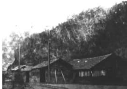
Original repair shop in Ibaraki (1910)
