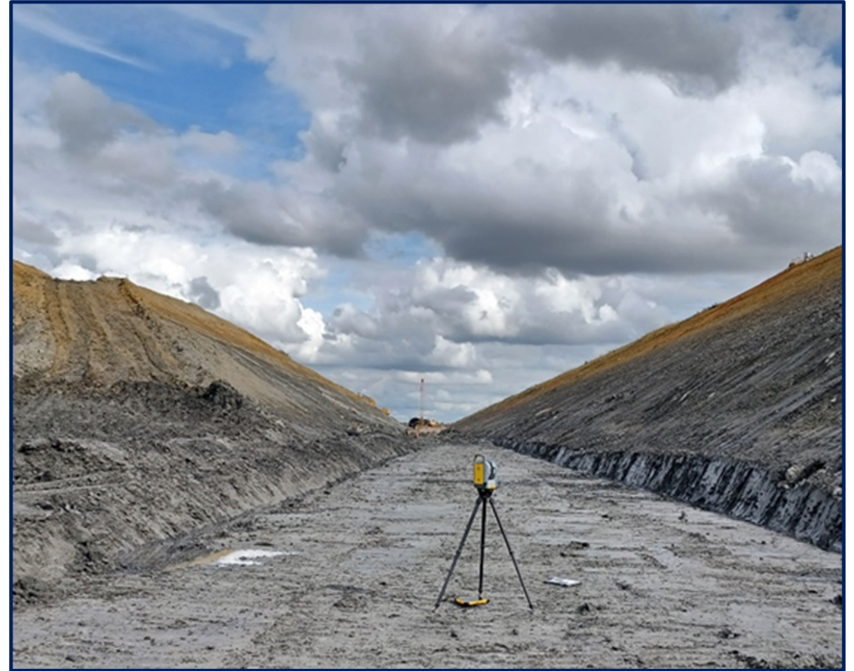
Trimble X7 3D laser scanner in cutting in mudrocks
