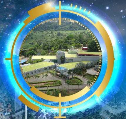
SATELLITE DATA RECEIVING STATION TEMERLOH, PAHANG
