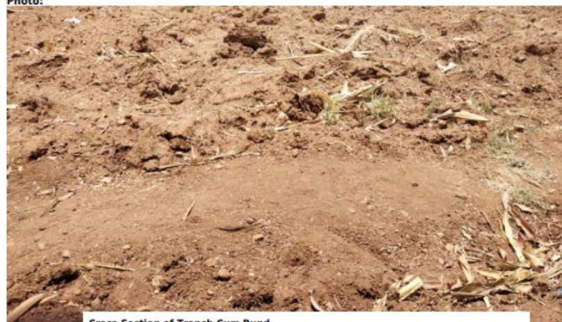
Cross Section of Trench Cum Bund
